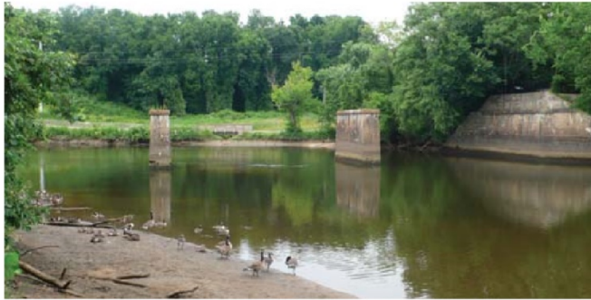
Existing bridge abutments
