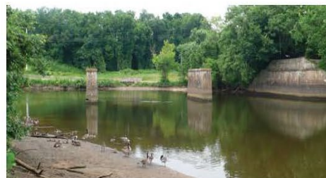
Existing bridge abutments
