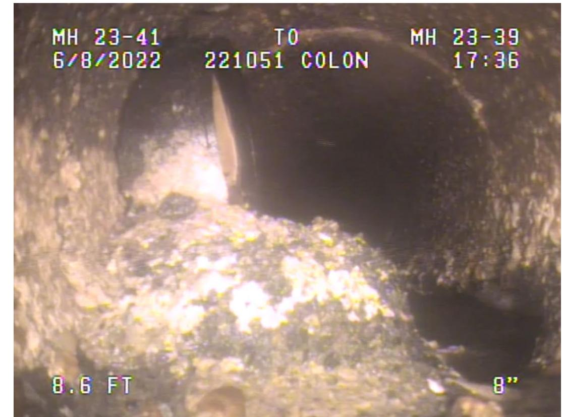
Level III: The pipe is fractured, offset, and broken. Point repair is required before installation of CIPP.
