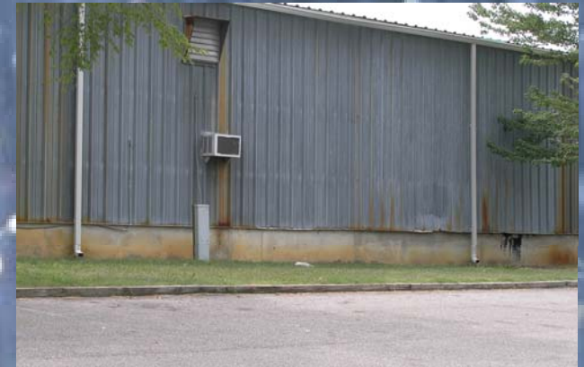
Downspouts contribute pollutants and to runoff velocity of stormwater
