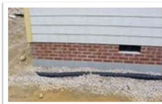
Foundation/Footing Drains
