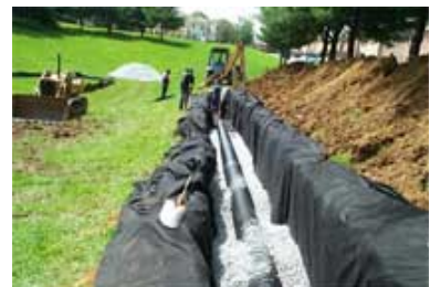
Infiltration trench under construction
